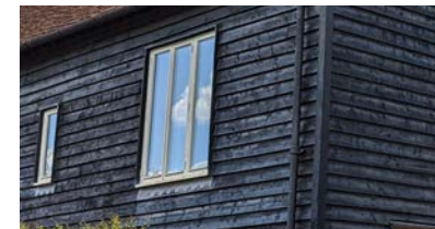
Modern windows on a converted barn
