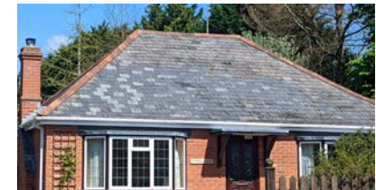
Grey slate tiles on a hipped roof
