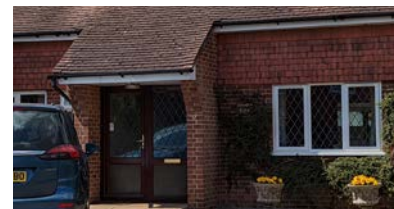
Porch under a catslide roof
