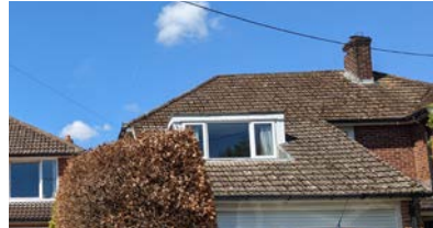
Clay tiles on a catslide roof
