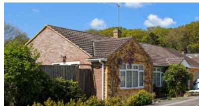
Clay tiles on a cross gabled roof
