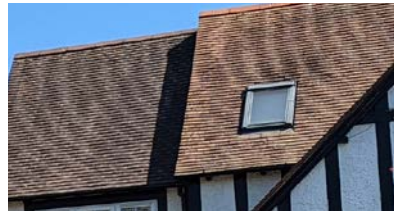
Red clay tiles on a gabled roof
