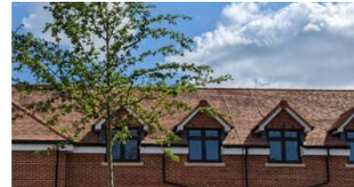
Red clay tiles on a gabled roof with gabled dormers
