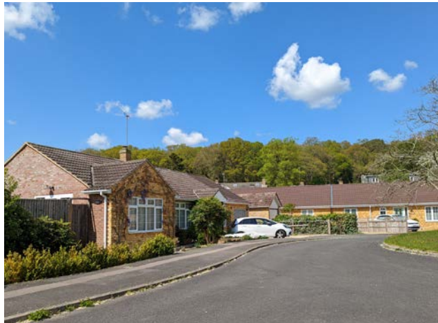
Figure 21: The rich backdrop vegetation is a characteristic of the village and it can be appreciate it to its fullest within low rise developments.
