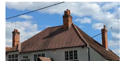
Hipped roof with red brick chimneys
