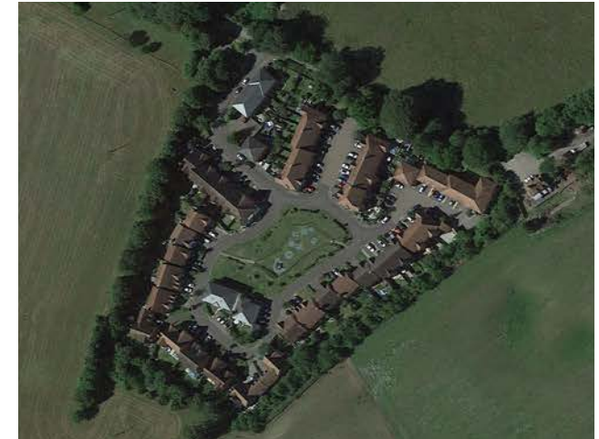
Figure 25: Local example of recent development in the village where properties back the open countryside with soft edges to mitigate any impact on the surrounding countryside, Hermitage Green.
