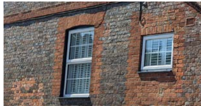
Sashed window framed with red brick
