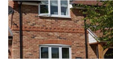
Buffed coloured brick with red brick details around the window frames
