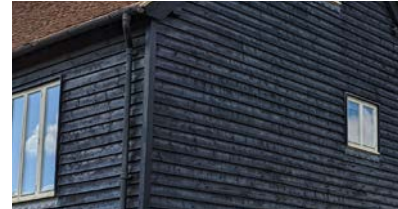
Horizontal dark weatherboarding
