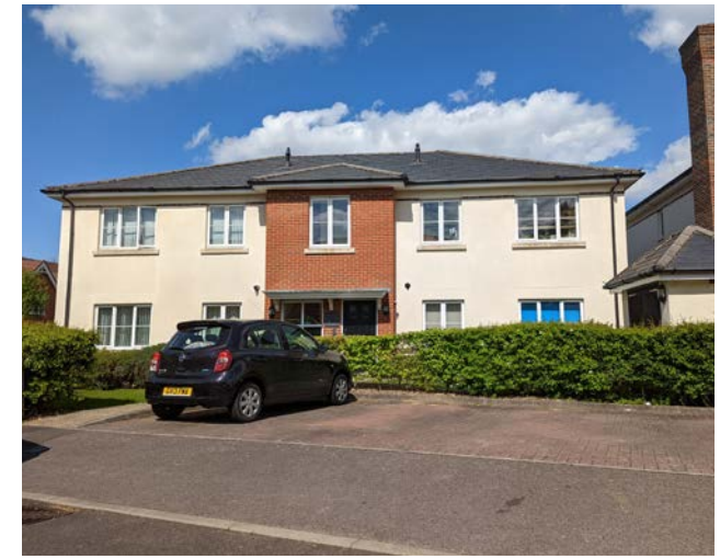
Figure 65: 2-storey flats located in Hermitage Green - example of local housing style.
