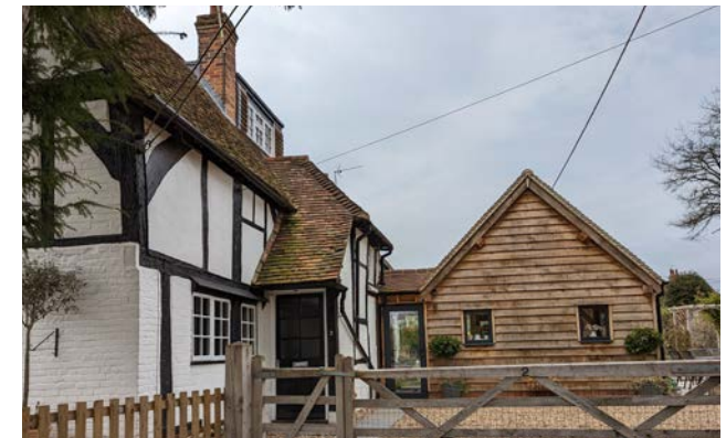
Figure 72: Positive example of a side extension that respects the existing building in terms of scale and building materials. In particular, the use of weatherboarding positively reflects back to the typical appearance of barns and outbuildings, elsewhere in UK.
