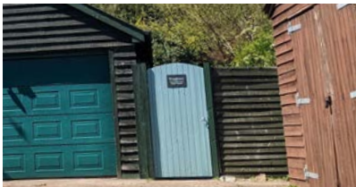
Timber door & horizontal timber fencing
