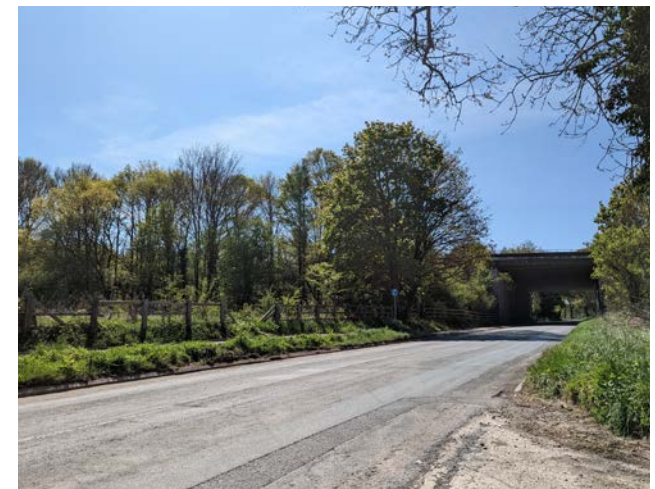
Figure 09: View to the spine road (B4009), towards the edge of the village settlement, where there are no pavements on either side and the road has a more rural character.
