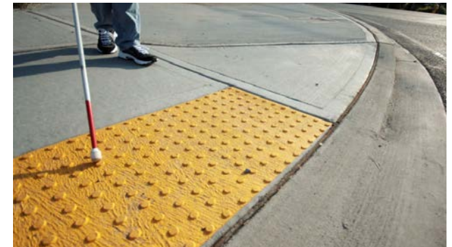
Figure 57: Example of tactile paving to facilitate movement for people with visual impairment.
