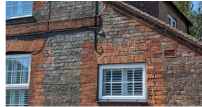
Variations of brick colour on facade
