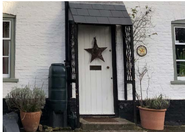
Figure 118: Examples of water butts used for rainwater harvesting in Reach, Cambridgeshire.
