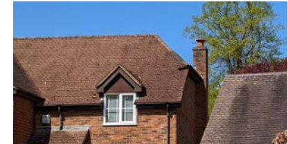
Red clay tiles on a mansard roof
