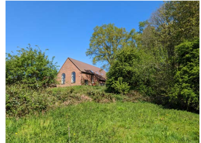
Figure 123: View to the Village Hall illustrating how rich the existing vegetation is within the parish.
