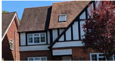
Timber frame with white render infills
